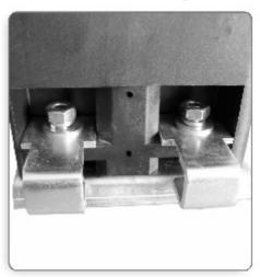
3. Re-fasten the washers and nuts to the retaining studs to secure the brackets.
